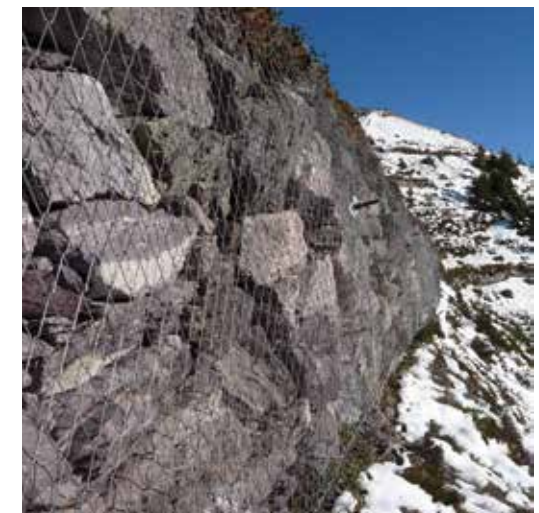
Fig. 11: Stone wall stabilized with anchored TECCO steel wire mesh (photo: M. Gächter)
