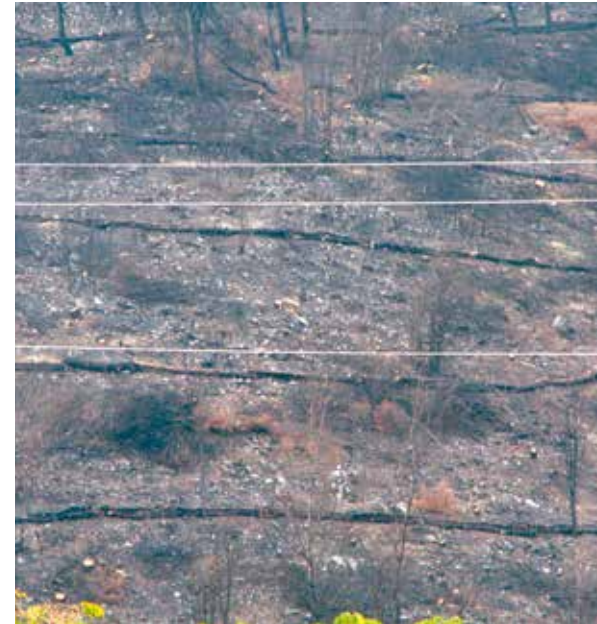
Fig. 3: Construction of Log Erosion Barriers
