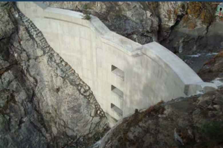
Abb. 1: Bogensperre in Stahlbeton. Fig. 1: Arched dam out of reinforced concrete
