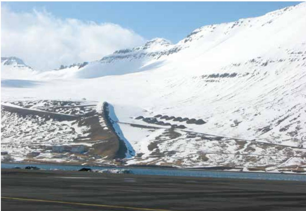
Fig. 4: The 16-m high deflecting dam on Seljalandsmúli in Ísafjörður, NW-Iceland. Two rows of breaking mounds have been built upstream of the dam to slow down the flow of the avalanche before it hits the dam (Photo: Tómas Jóhannesson, 16 April 2006).
